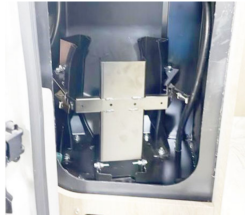
Propane Gas Access (Located behind the drivers side rear door behind the LP access door). -Typical View
