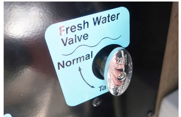
Fresh Water Valve (Shown in the open position. Turn valves to close). This is on the T36A and T36B -Typical View
