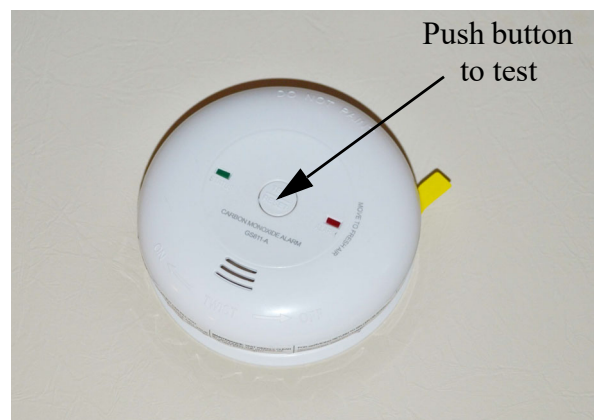
Carbon Monoxide Alarm
